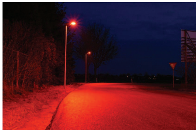
Figure 21: Red, bat-friendly streetlights along the A4440 have less adverse impacts than white lights (by Worcestershire County Council)
