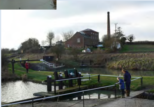
Wilton Water with canal & pumping station behind
