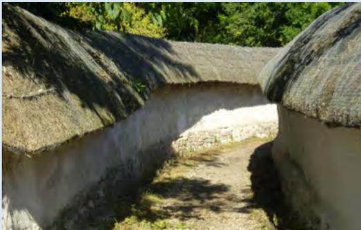
Lime-washed cob walls at Blewbury, protected from the weather by a thatch capping and rising damp by a stone base.
