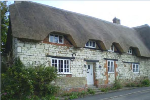
Chalk block cottage with brick and sarsen foundations and wooden lintels, Ashbury. Such chalk block cottages have resisted the weather for centuries by having “good shoes and a hat,” that is a plinth of stone or brick to stop rising damp and overhanging eaves of thatch to resist the weather.
